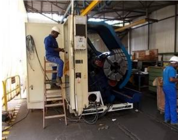
Figure 24: Alberto prepares the installation. WU_232_180
