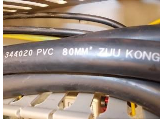
Figure 26: cable 80 mm / 2. Since the machine is operated in the country of origin to 115/220 volts, these thick cables are required. WU_232_200
