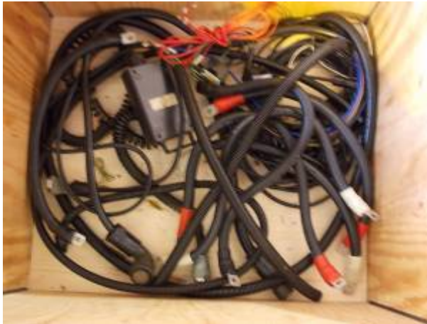
Figure 8: Removed old Fanuc cable. WU_232_80
