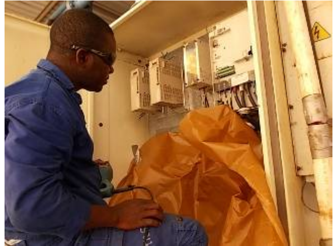
Figure 30: We had to explain to the boys when they do not cover the drilling, there can be a blast on power. Why must everything always be off-covered when drilling. WU_232_240
