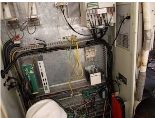
P25) Soon, everything installed fine and it still has a little vacant position.
