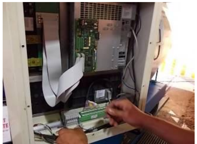
P29) The fact is, there are significantly fewer cables that hang around there. Surely only 30%. Optical and much more pleasant to use.
