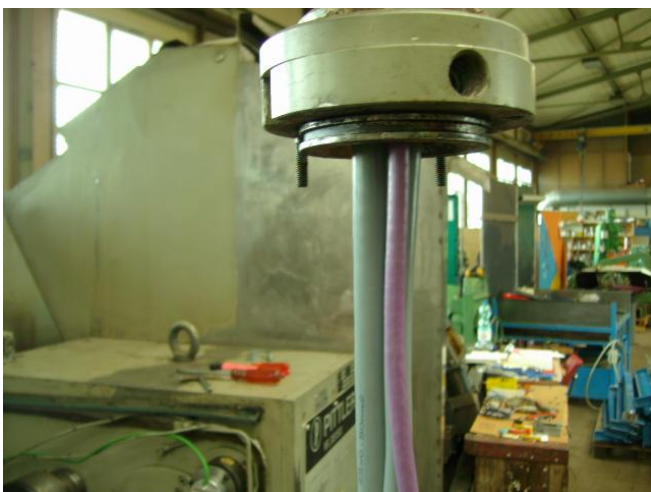
Figure 12: The old panel suspension could well be used again for the new CNC. Very stable.
