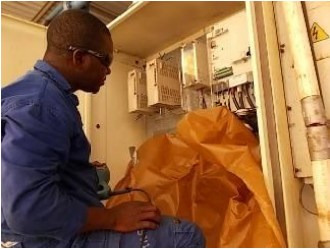
P24) We had to explain to the boys when they do not cover drilling, there may be a pop when turning because chips are not allowed in the electricity and electronics. That's why everything has to be covered when drilling.
