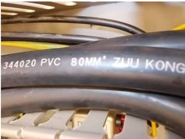
P20) Since there are cables with 80 mm / 2. Since the engine is operated in the country of origin 115/220 volts, this thick cables have been installed.
